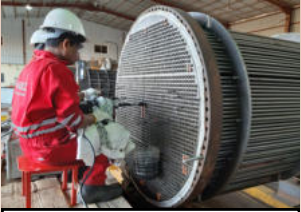
HEAT EXCHANGER RETUBING
