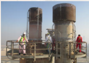
FLARE REPLACEMENT / REPAIR
