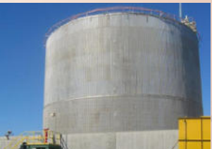
TANKS & VESSELS MAINTENANCE
