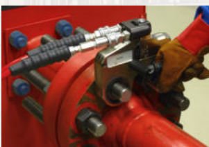
BOLT TORQUING & TENSIONING
