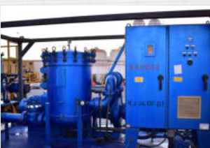
LUBE OIL FLUSHING & FILTRATION
