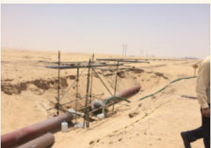
PIPELINE FABRICATION / ERECTION
