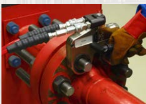
BOLT TORQUING & TENSIONING
