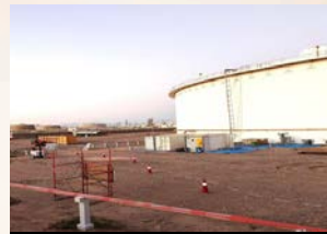
AUTOMATIC TANK CLEANING (ATC)
