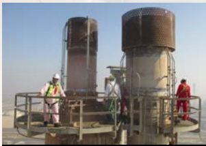
FLARE REPLACEMENT / REPAIR
