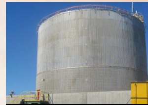
TANKS & VESSELS MAINTENANCE
