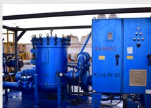
LUBE OIL FLUSHING & FILTRATION
