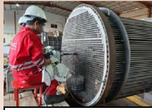
HEAT EXCHANGER RETUBING
