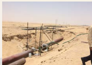
PIPELINE FABRICATION / ERECTION
