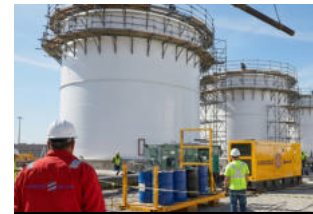
TANKS & VESSELS MAINTENANCE
