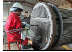
HEAT EXCHANGER RETUBING
