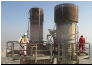
FLARE REPLACEMENT / REPAIR
