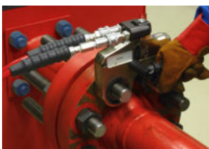
BOLT TORQUING & TENSIONING
