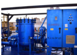
LUBE OIL FLUSHING & FILTRATION
